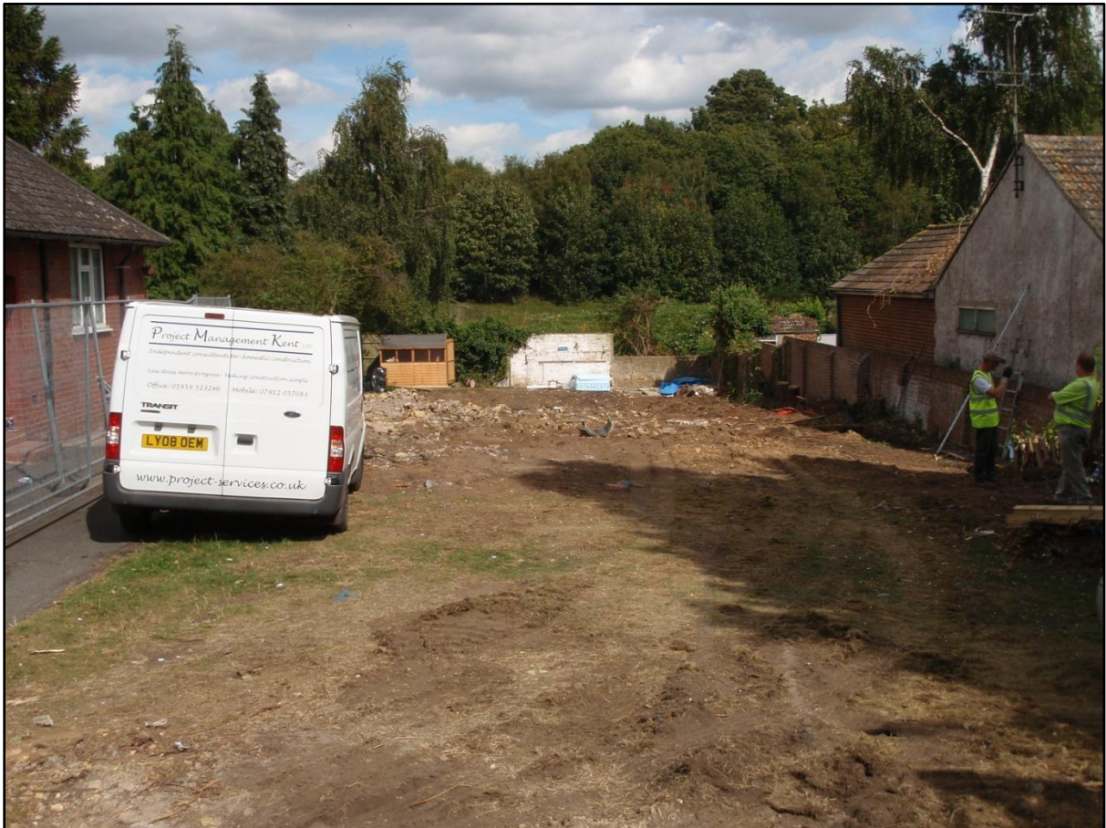
Plate 2. General view of site prior to ground works facing north
