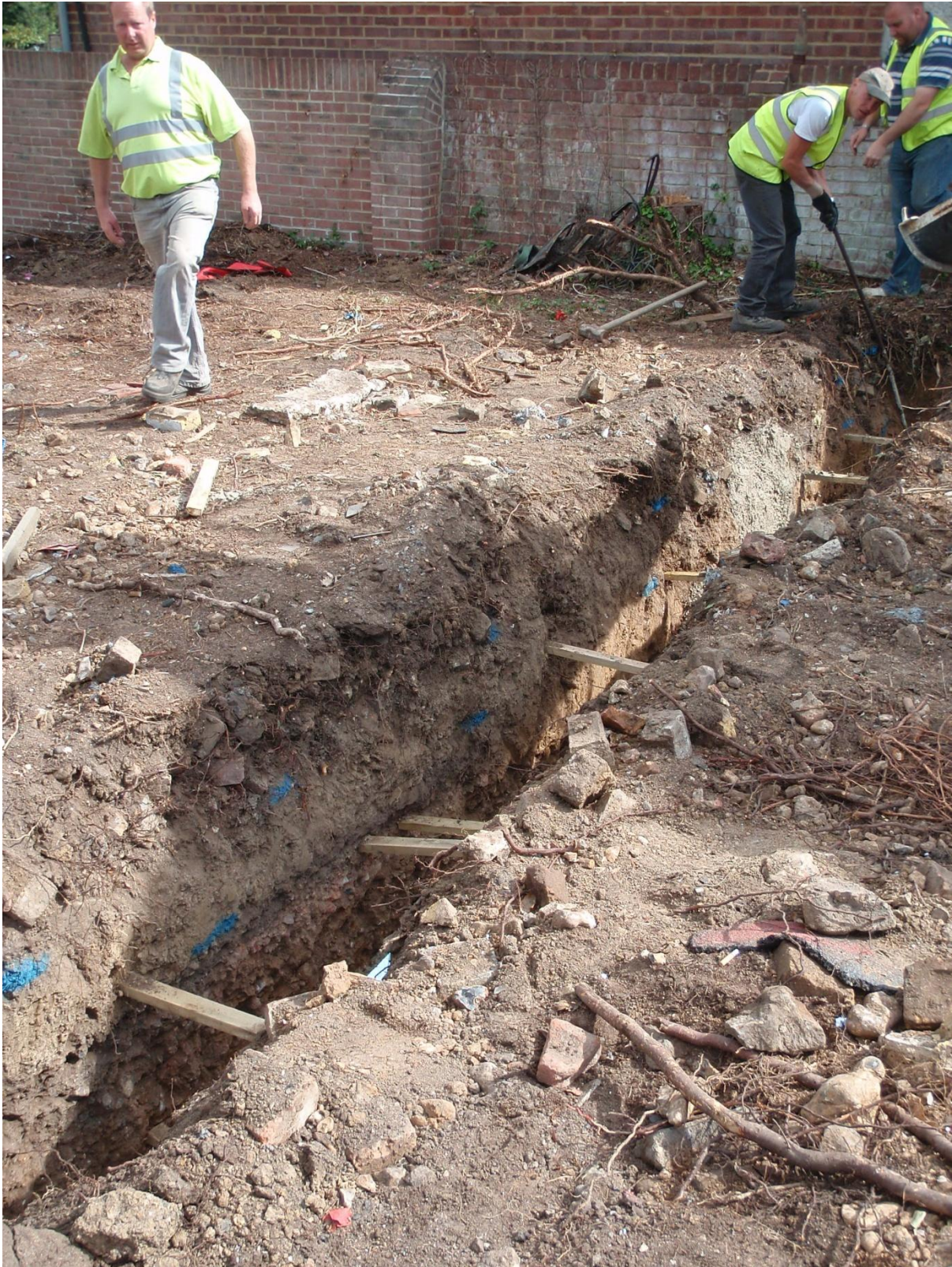
Plate 3. The site showing overburden of topsoil mixed with demolition material
